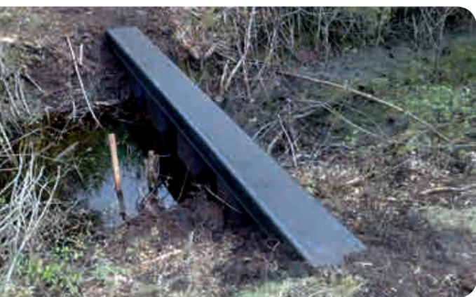
Sheet piling in drainage ditch
